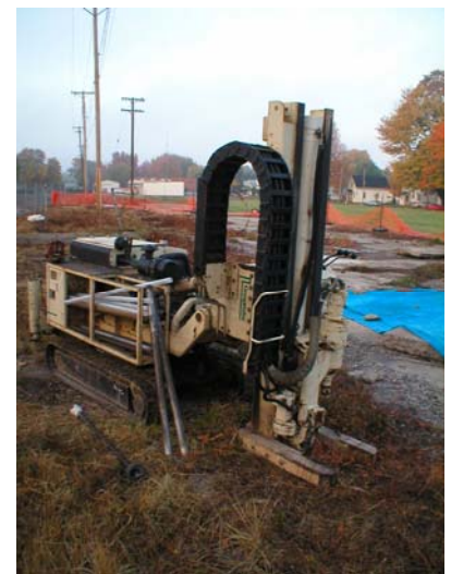
Direct-Push Drilling Rig
